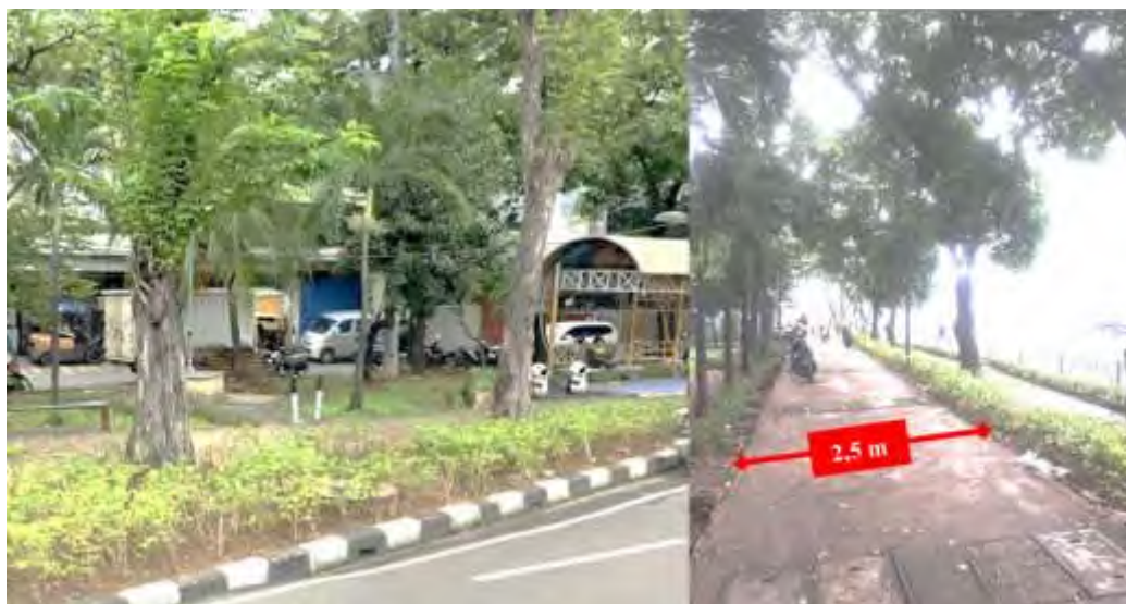
Figure 2. Existing condition of the study area.
