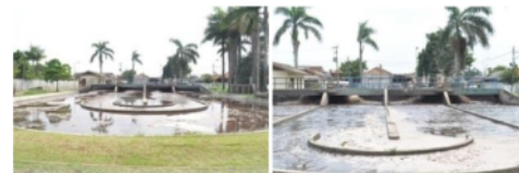
Figure 3 Oxidation ditch unit in WWTP Tanah Tinggi [12]
