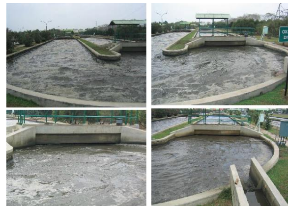
Figure 2 Oxidation ditch unit in WWTP Jababeka [11]
