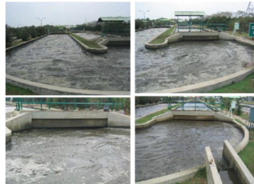
Figure 2 Oxidation ditch unit in WWTP Jababeka [11]
