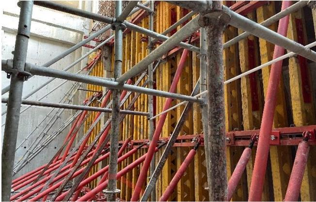
Gambar 27 Pemasangan Bekisting Dinding
