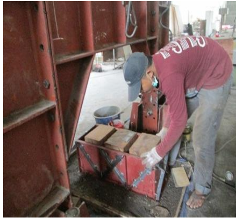
(a) Panel beton polystyrene didiamkan selama 24 jam
