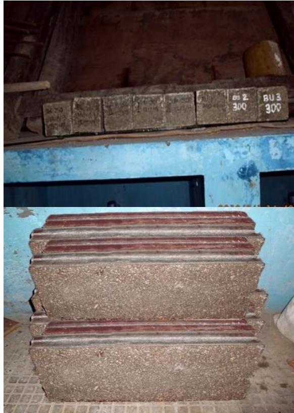
Gambar 4.23. Tahap perawatan beton polystyrene
