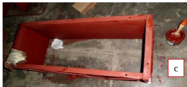
(c) Bekisting plat
