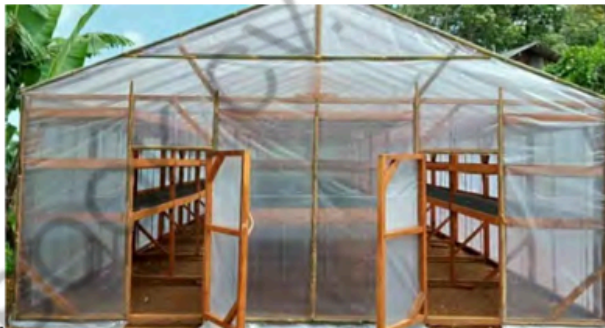
Gambar 32. Green house di Pangandaran Gugi Samugya (Ruber, 2020)
